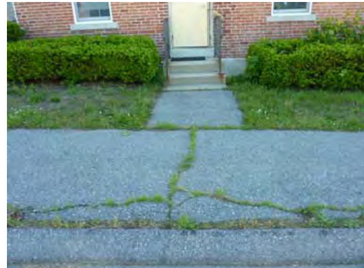
Typical cracking of asphalt paving at walks; trip hazard at first riser at concrete stoop is shown to be eliminated in Year 1.
