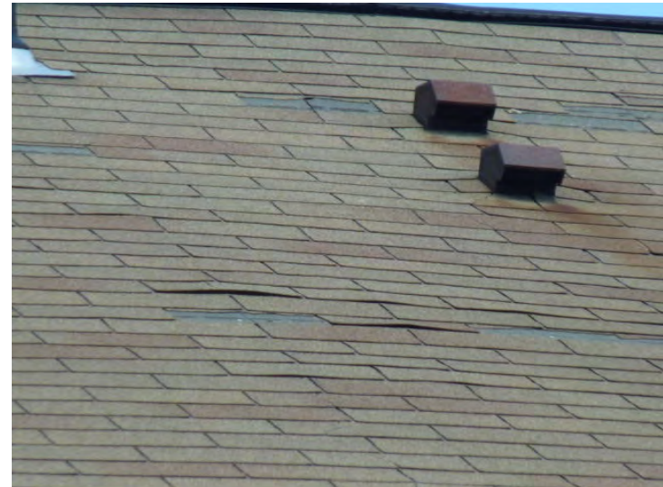
Lifted and missing shingles at 29 Tiffany Place to be replaced in Year 1.
