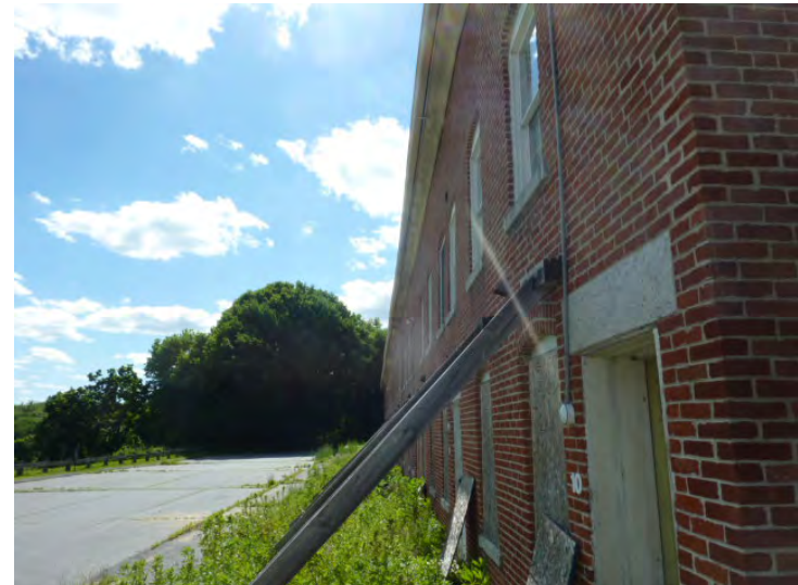
Rear wall at 5 Front Street is bowed along lateral bearing line of lateral braces.
