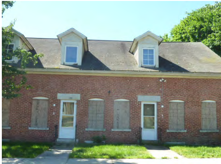
Worn roofing at 5 Front Street to be replaced and dormers repaired and painted in Year 1.
