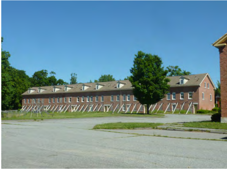
Lateral bracing along 5 Front Street building installed to stabilize wall due to the wide spacing of original lateral ties that exceeds allowable spacing.
