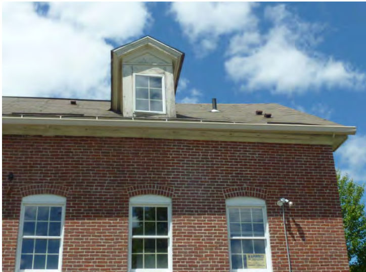
Warped roof at end bearing wall at 29 Tiffany Place.
