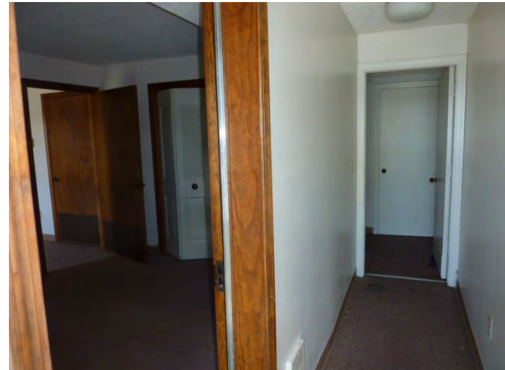
Door to second floor unit on right and door to two-bedroom flat on left at 5 Front Street. Fire rated frames and doors are shown for Year 1.
