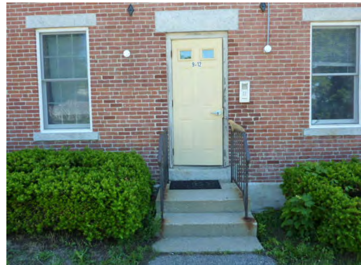
Trip hazard at concrete stoop and rusted handrails shown to be eliminated in Year 1.
