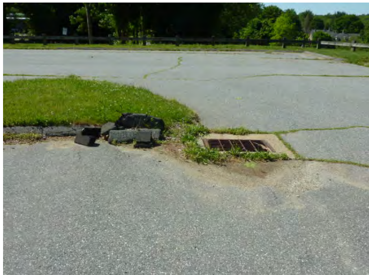
Current damage to asphalt curb and historic settlement at catch basin.
