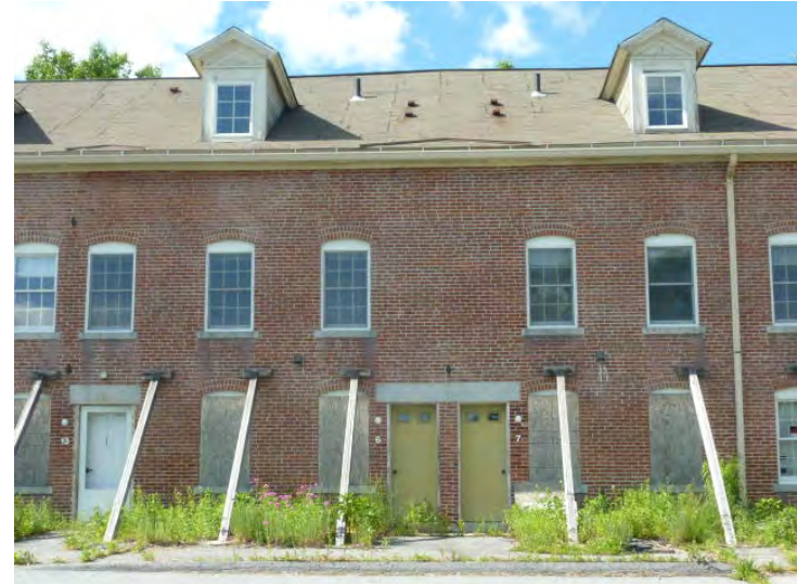
Roof framing and shingle roof is bowed on both sides of bearing wall between pair of yellow doors at 5 Front Street.
