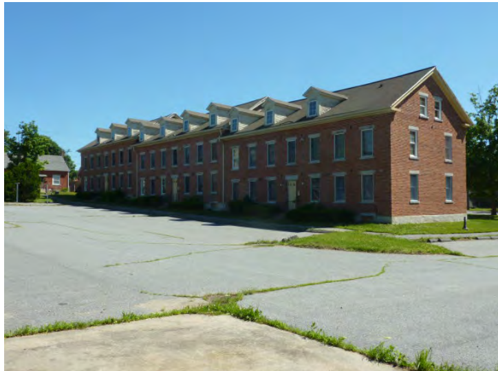
Typical cracking of asphalt paving at parking lots behind 29 Tiffany Place.
